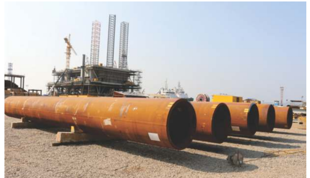
Execution of the contract for provision of SVSW Piles and Conductor Piles Manufacturing Service for PTSC M&C under the Southwest Golden Lion Project
