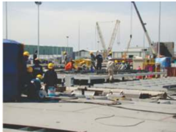
PVSB's workers fabrication and installation of mechanical engineering oil and gas safety
