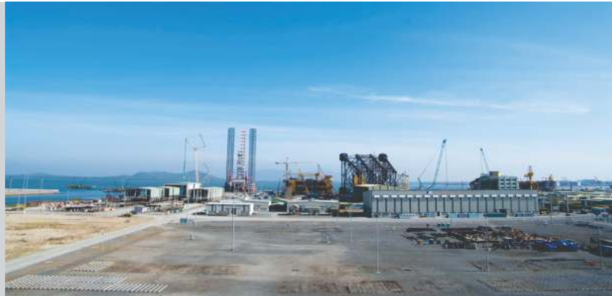
Ground infrastructures are leased to PVShipyards in Sao Mai – Ben Dinh Petroleum Marine Service Base
