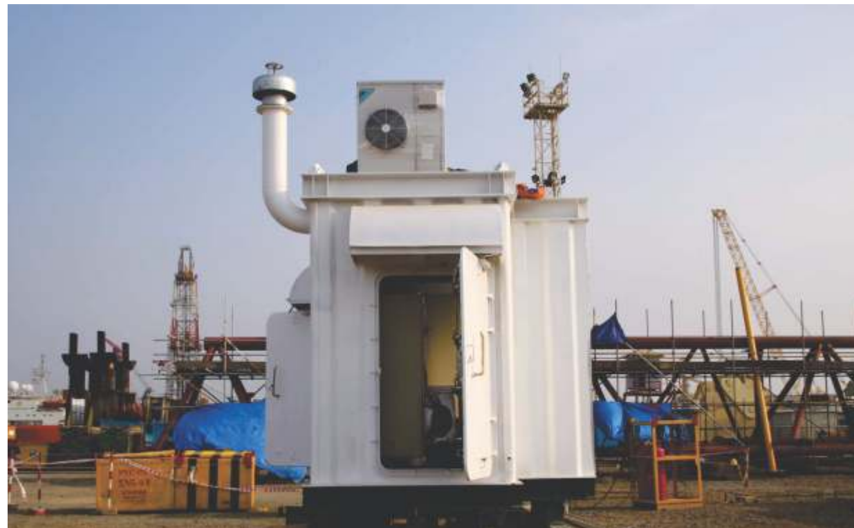
On 22/1/2015; at construction site of Vietsovpetro's offshore construction division, Representative of Sao Mai – Ben Dinh Petroleum Investment JSC, VSP and DNV Register have held a ceremony to sign the acceptance minutes of UPS & Battery room under Contract No. 0190/12-XL1 / PVSB
