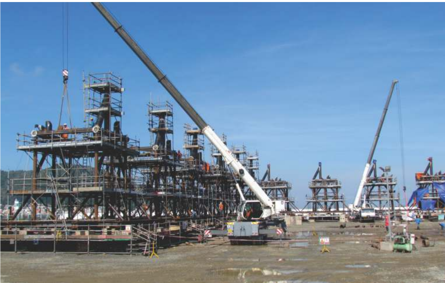
Workers of the Company are constructing, manufacturing and installing the petroleum mechanical work at the Site
